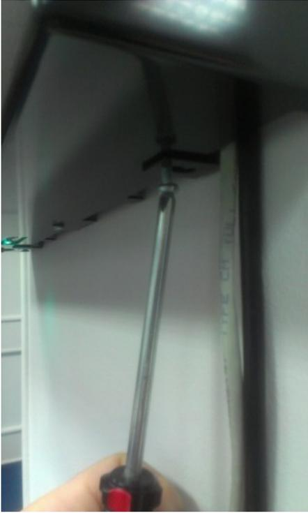
Now it's time to hang the screen. As a default, you can either have the wiring come from behind or route it through the vent slots at the bottom of the unit (as shown opposite). If you want to have top-entry, there are a pair of press-out sections of the case that can be removed as required by wiggling with a pair of pliers.
