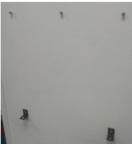
Fit the screws - drive the top ones in first. The exact depth will depend on the fixings you use, but aim to leave 3-4mm of shaft exposed to allow the screen case to hang off them.
